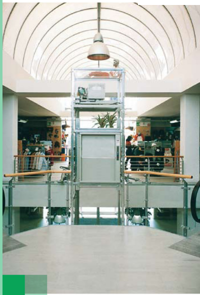
Installation in a clothing shop, model 50 kg, glass cladding and standard bar in RAL 7038.
